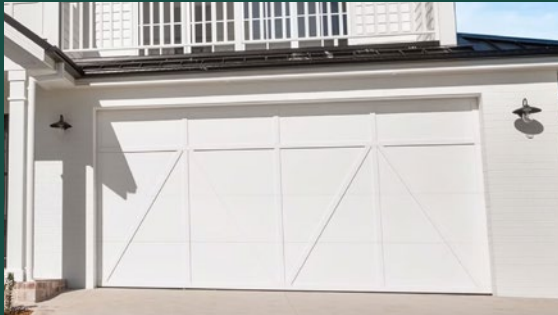
DETAILED DOOR WITH CONCRETE DRIVEWAY
