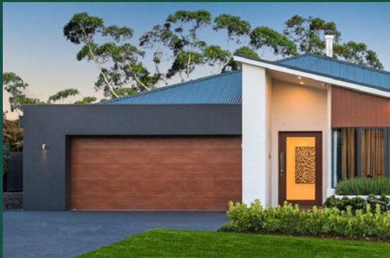
SECTIONAL DOOR WITH CONCRETE DRIVEWAY
