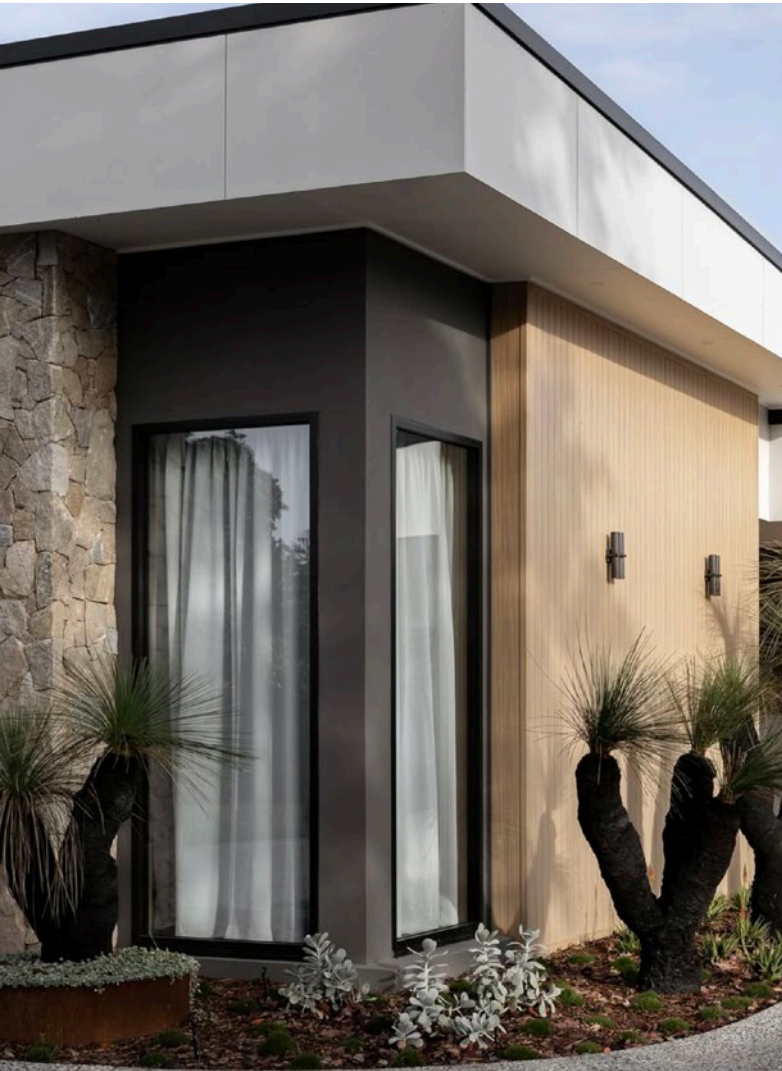
Source: Cook Constructions
