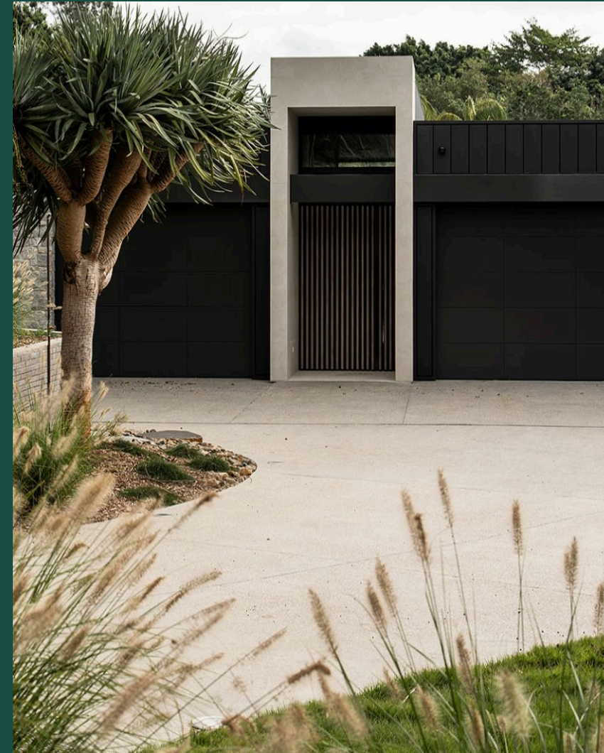
SECTIONAL DOOR WITH CONCRETE DRIVEWAY
